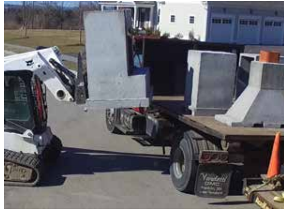
Step 2: Units are delivered to job site.
