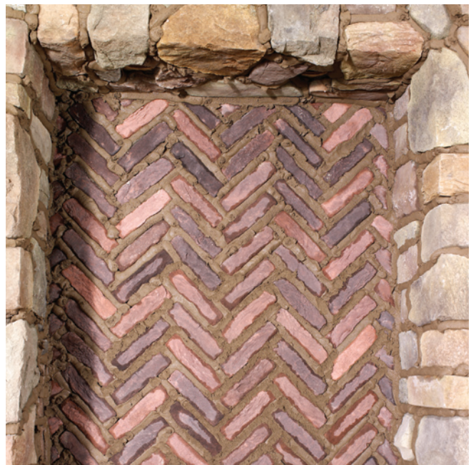
Above: Smooth the mortar flush with face of brick. Above right and below: Overlapping face of brick creates desired rustication.
