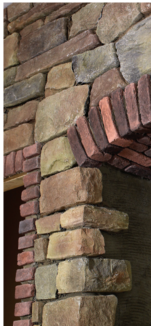
Above and below left: Install brick first using chalk lines and level. Below right: Alternate stone corners so returns vary.
