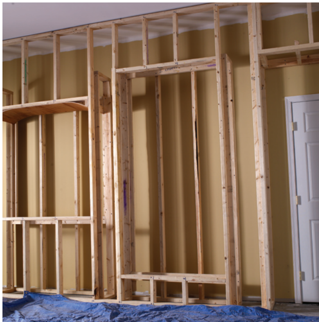
2 x 4 construction creates the needed depth
