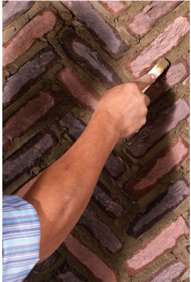
Above: Smooth the mortar flush with face of brick. Above right and below: Overlapping face of brick creates desired rustication.
