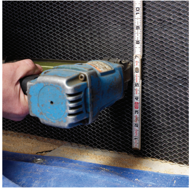
Attach lath with galvanized nails or staples.
