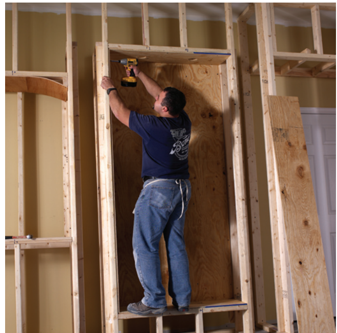
Locate supports where necessary
