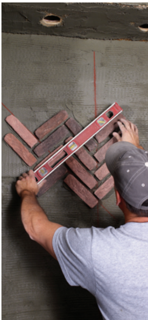
Above and below left: Install brick first using chalk lines and level. Below right: Alternate stone corners so returns vary.
