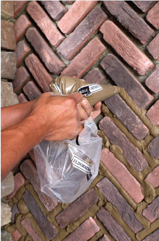
Above: Smooth the mortar flush with face of brick. Above right and below: Overlapping face of brick creates desired rustication.
