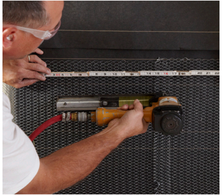
Attach lath with galvanized nails or staples.
