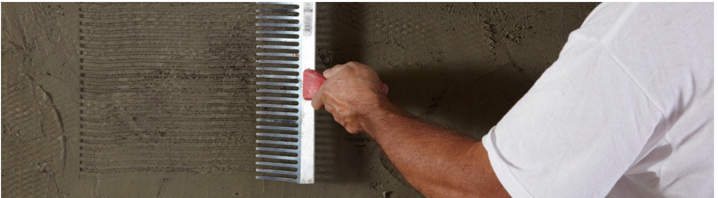
Cover entire lath with mortar and score mortar horizontally.
