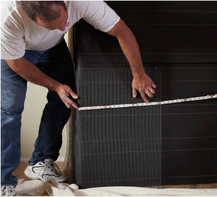
Install weather-resistant barrier and metal lath.
