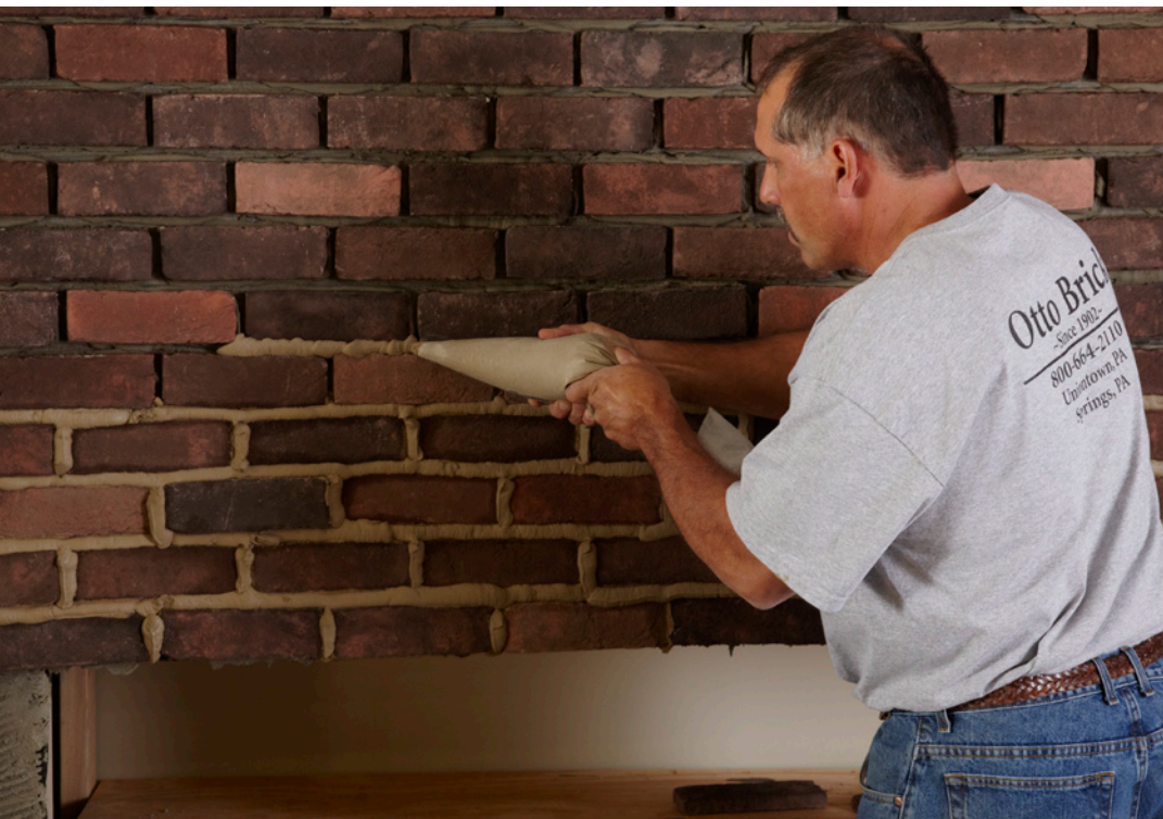
Adding color to the mortar can create an attractive combination.
