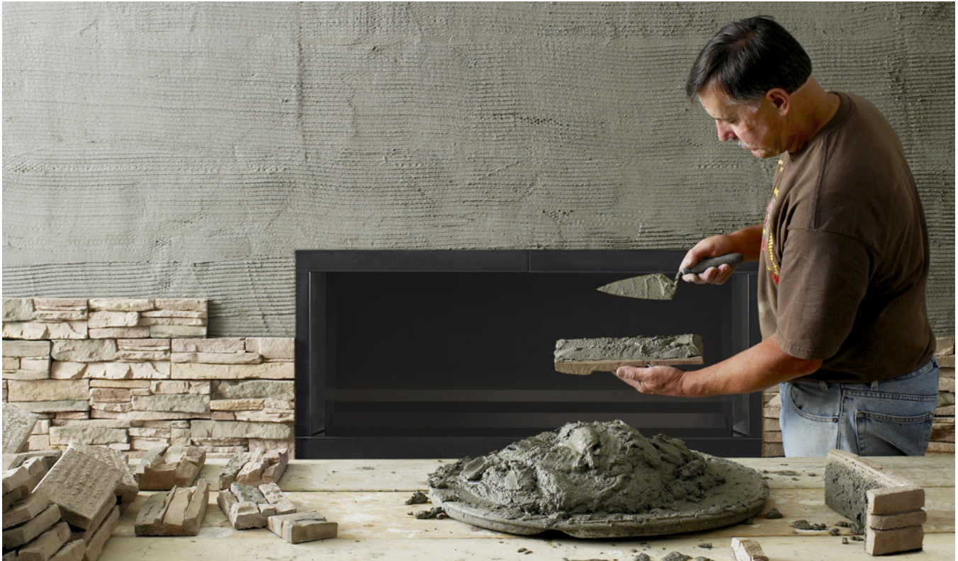
Apply a layer of mortar to back of veneer. Install corner stones first then straight stones. Consult eldoradostone.com for detailed installation instructions.
