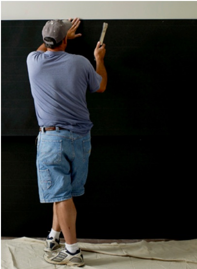
Install weather-resistant barrier.
