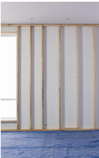
Wood stud framing over existing wall, location of candle niches and ply-wood sheathing.
