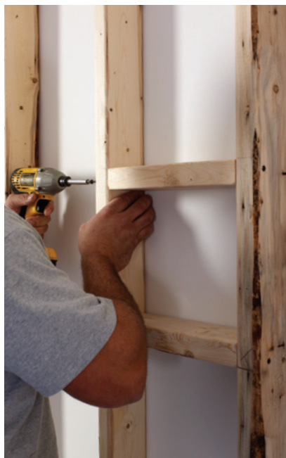
Wood stud framing over existing wall, location of candle niches and ply-wood sheathing.
