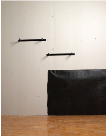
Install weather-resistant barrier.
