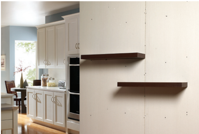
Placement of the shelving brackets and shelves prior to stone installation so shelves appear recessed within the stone upon completion of ArtWall.
