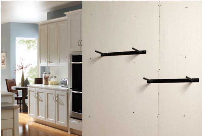
Placement of the shelving brackets and shelves prior to stone installation so shelves appear recessed within the stone upon completion of ArtWall.
